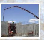
23,074 cubic yards of concrete and 265 tons of structural steel were used in construction of the plant, as well as 195 miles of electrical wire.
