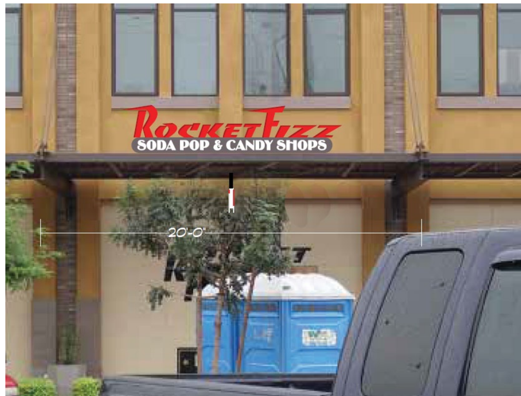
Canopy Mounted Sign With Integrated Raceway
