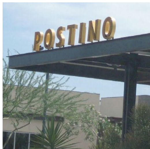
Illuminated dimensional letters mounted on canopy Allowable Tenant Sign Configurations Photos are examples only
