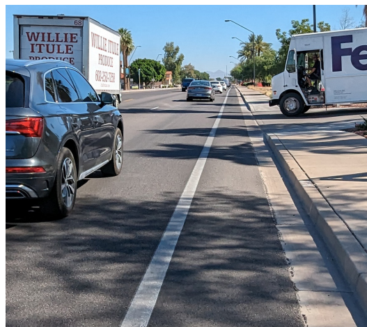
Figure: North bound on Gilbert Rd S of Rawhide Ave
