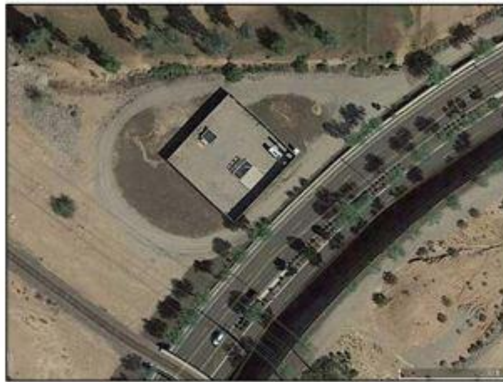
Photo 57 – Crossroads Pump Station Aerial
