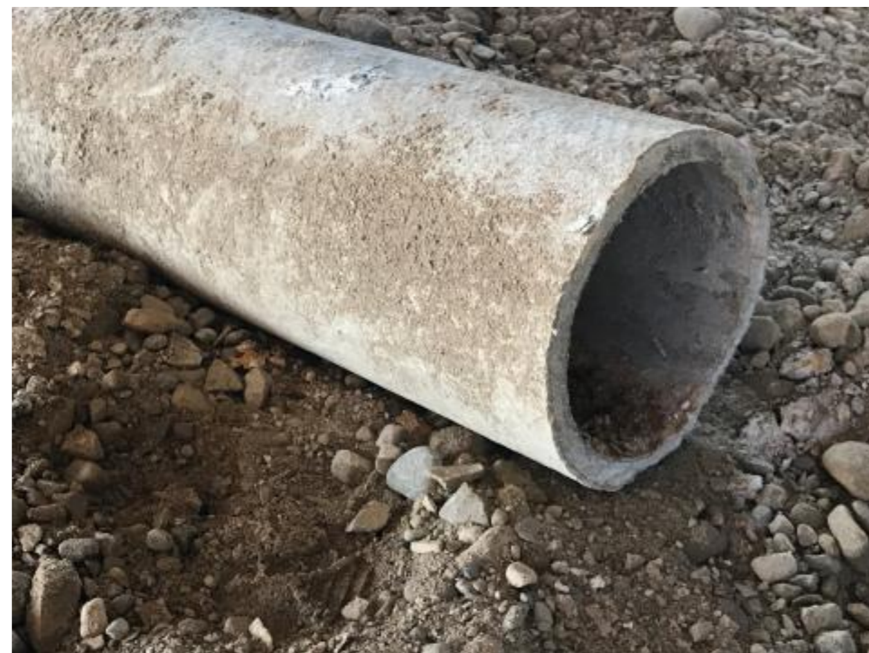
ACP (Asbestos-Cement Pipe) approximately 10%
