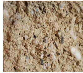
SPLIT-FACE CMU BLOCK OFFICE "PISMO DUNES"
