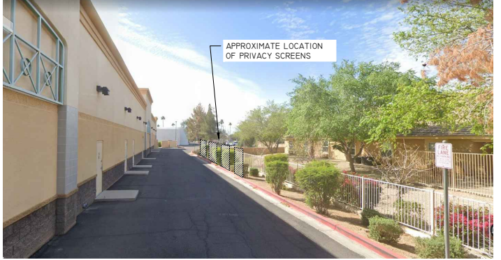
2 EXISTING REAR ALLEY
