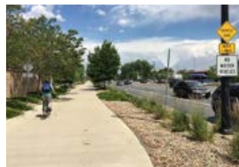
A wide shared-use bikeway allows plenty of room for passing bicycles and for pedestrians.
