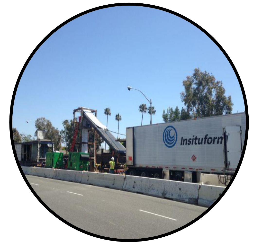
Cured-In-Place Pipe Lining (CIPP)
