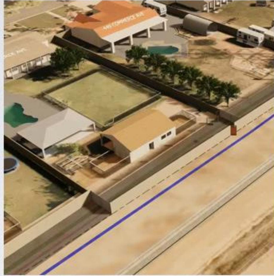
Utility Corridor Alley
