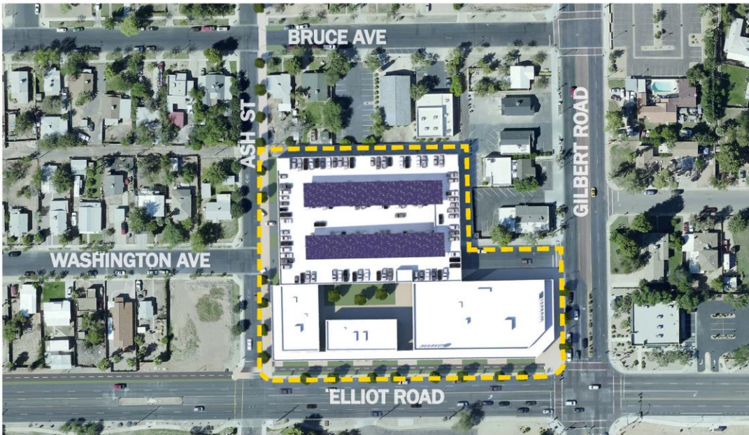
South Anchor - After
