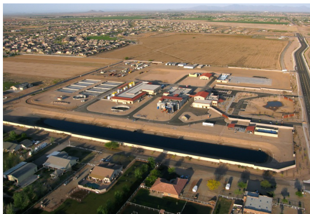
Santan Vista Water Treatment Plant
