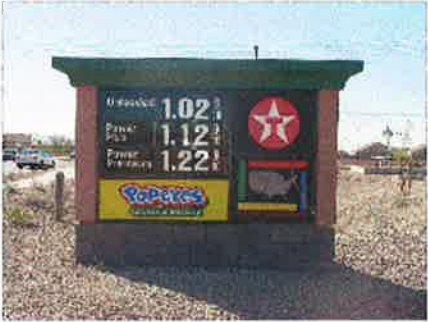
① EXISTING MONUMENT SIGN AND BASE ALONG VAL VISTA ROAD SCALE N.T.S.
