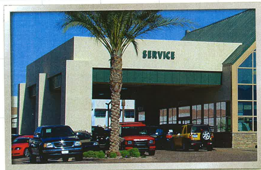
TERTIARY TYPICAL BUILDING SIGNAGE
