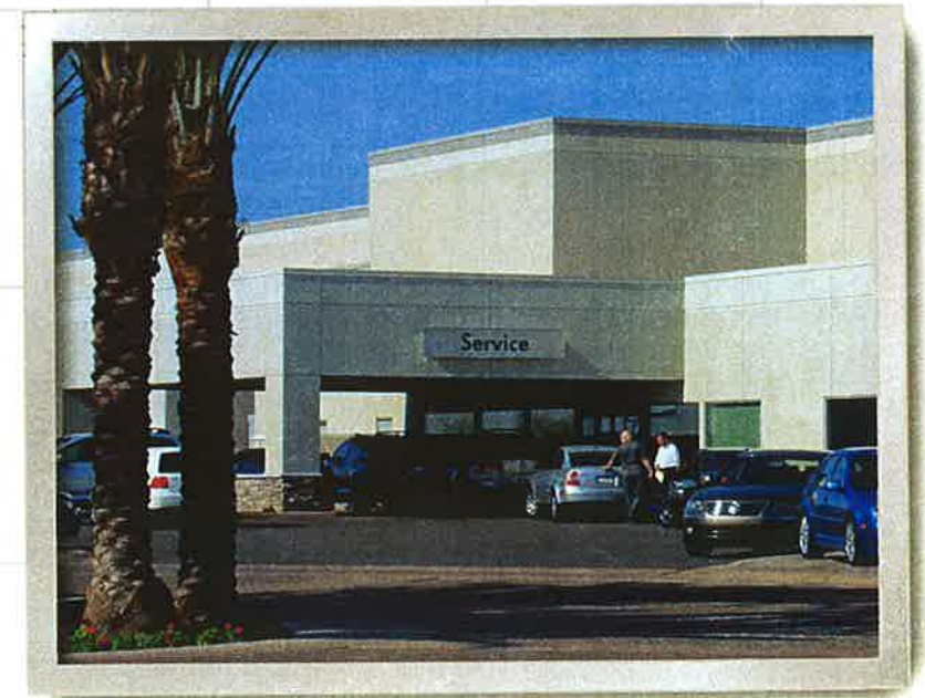
TERTIARY TYPICAL BUILDING SIGNAGE
