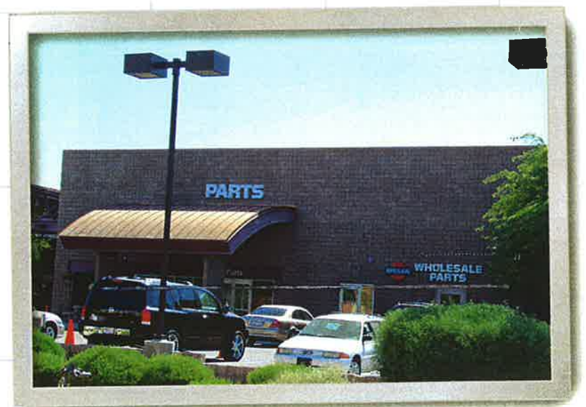
TERTIARY TYPICAL BUILDING SIGNAGE
