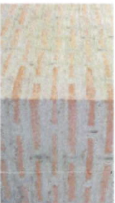
23 Brick with Mortar Wash
