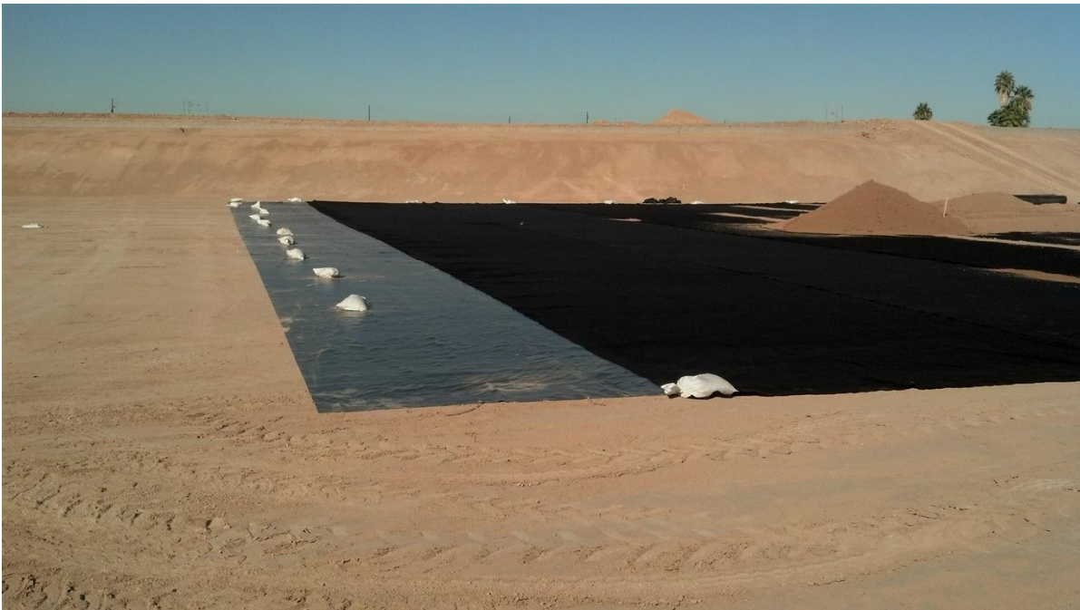
PVC Liner Installation at Pioneer Park in Peoria, Arizona
