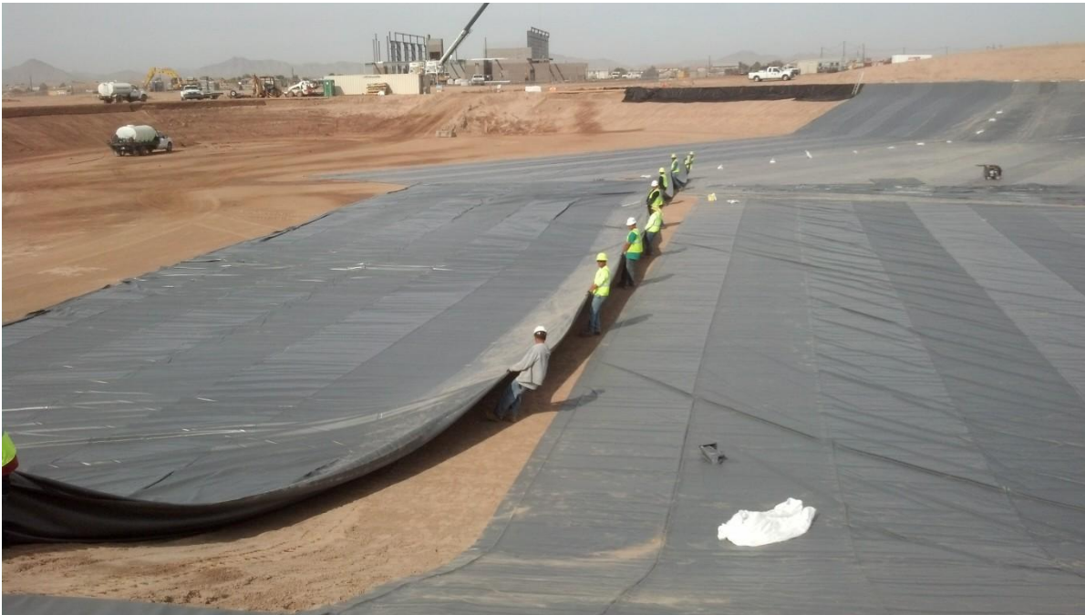
PVC Liner Installation In-progress at Copper Sky Park in Maricopa, Arizona
