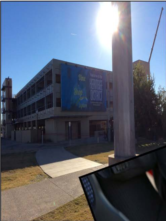
Vaughn Avenue Parking Structure in the Heritage District
