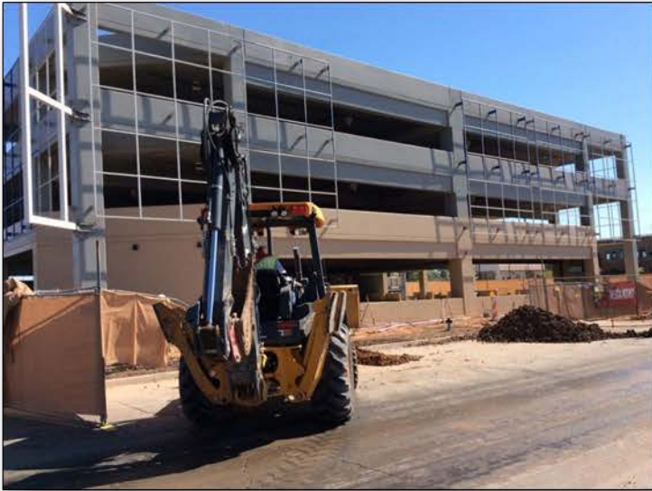
Vaughn Ave Parking Structure Capital Project # RD110
