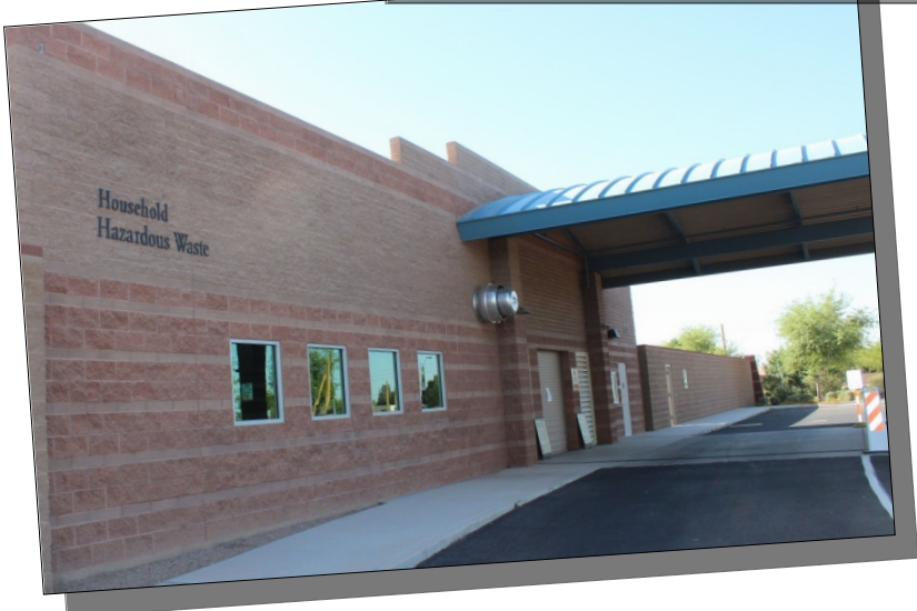
Environmental Services - Household Hazardous Waste Facility
