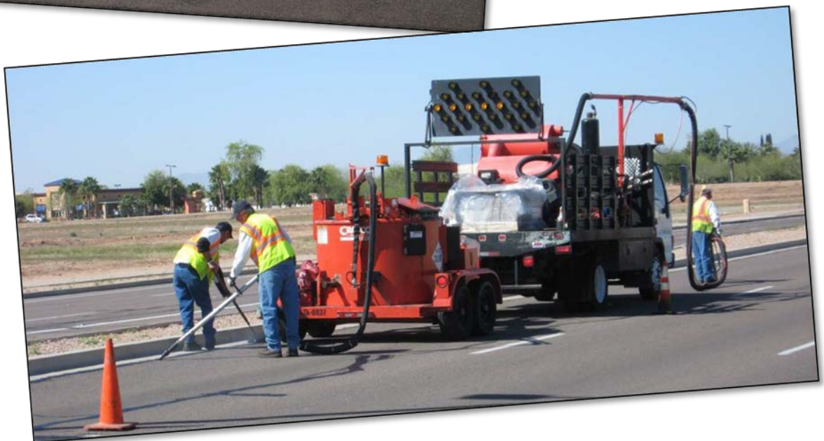
Performing preventative maintenance – crack seal team
